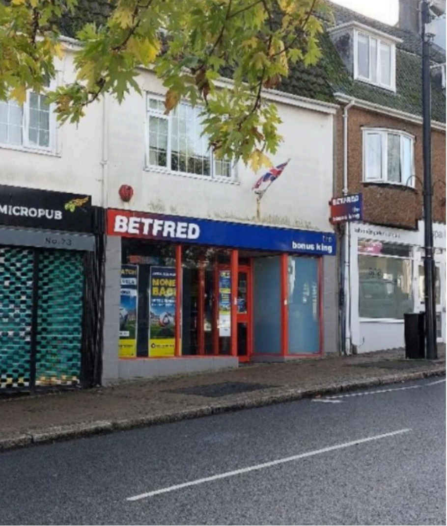
EXISTING : Description: Old flagpole above BETFRED commercial unit.
